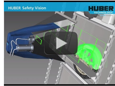
Animation: HUBER Safety Vision system for impurity detection
