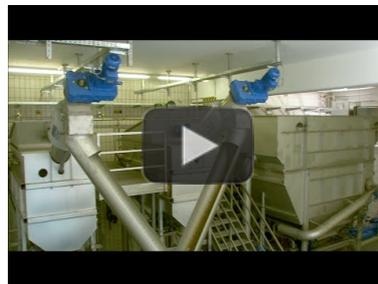
Video: HUBER Rotary Drum Fine Screen ROTAMAT® Ro2 for preliminary wastewater treatment in meat processing industry
