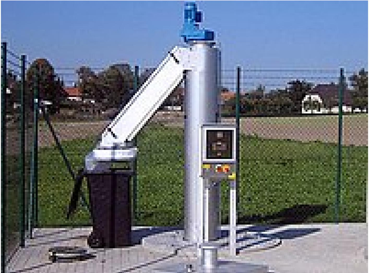
Automatically cleaned fine screen with vertical lifting, dewatering and compaction of screenings
