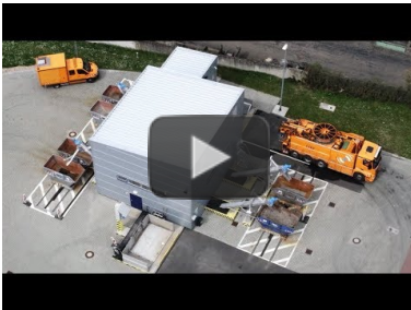
Video: HUBER ROTAMAT® Wash Drum RoSF9 in a grit treatment process for coarse material separation
