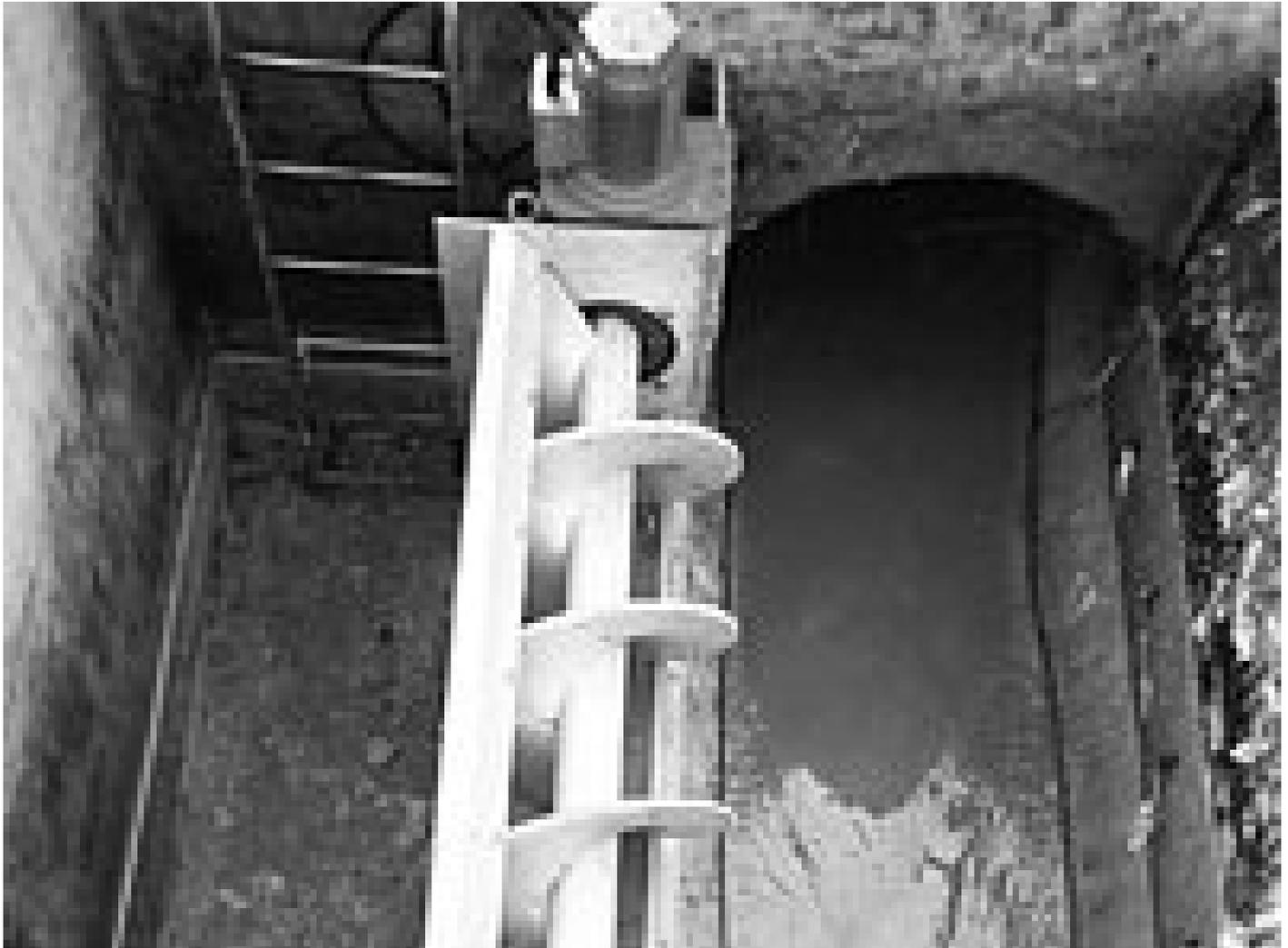
*Screening of up to 10 m<sup>3</sup>/s combined water with 6 mm perforated plate*
