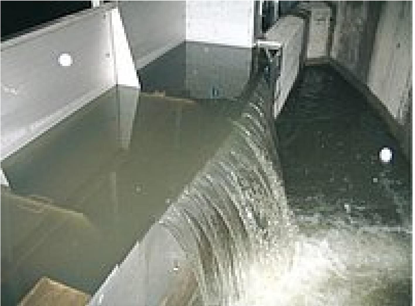
*Sewage flowing through our RoK 2 screen and overflowing our measuring weir*
