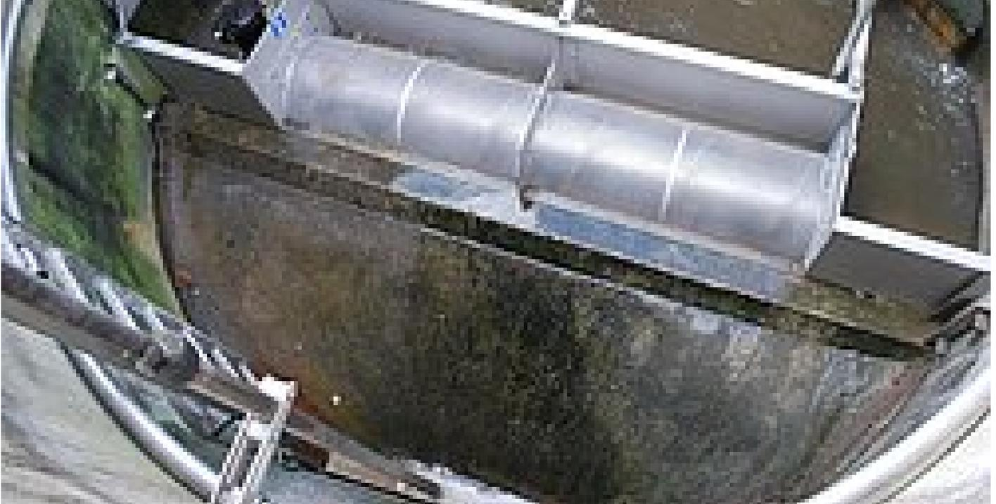
*HUBER Storm Screen ROTAMAT® RoK2 in a stormwater overflow structure*
