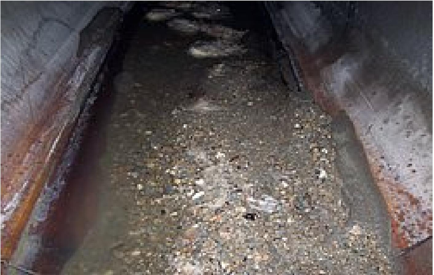
*Sediments in a combined sewer after a longer dry weather period*
