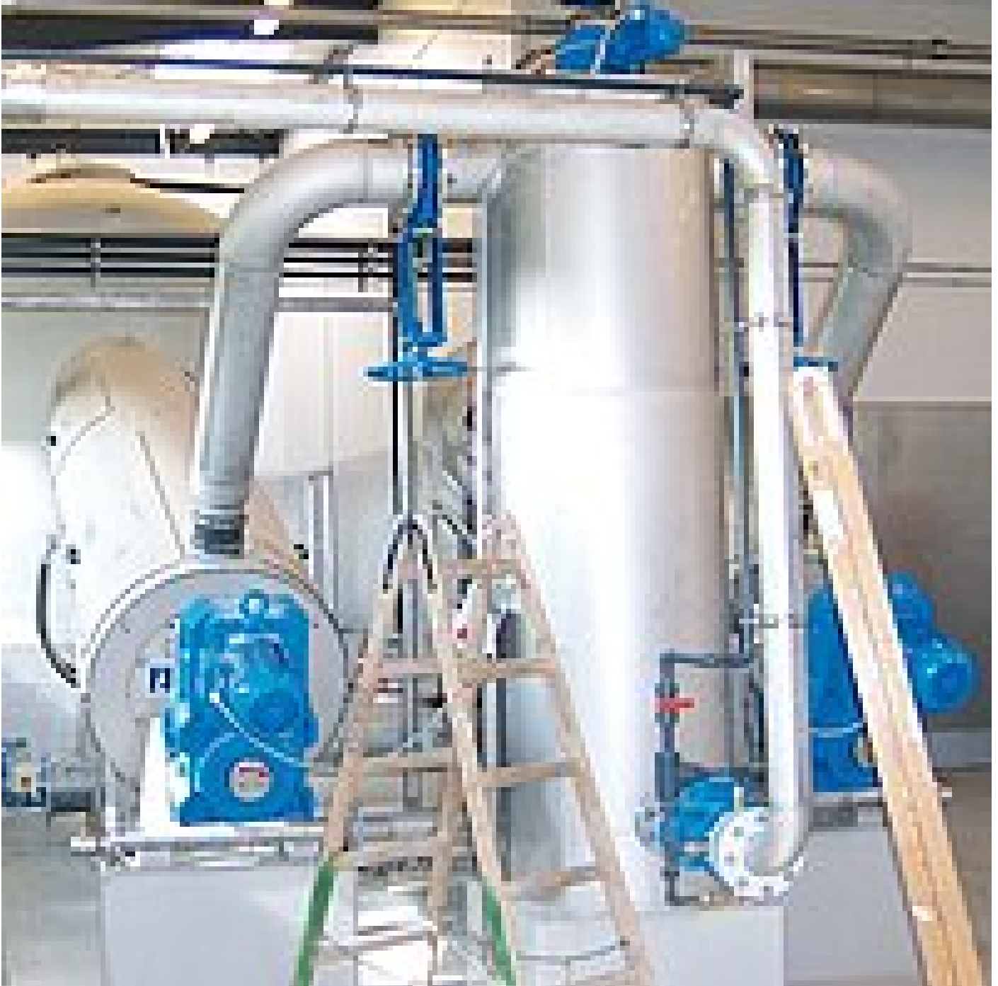
ROTAMAT® RoS 3/3 for flotante sludge dewatering with flocculation reactor
