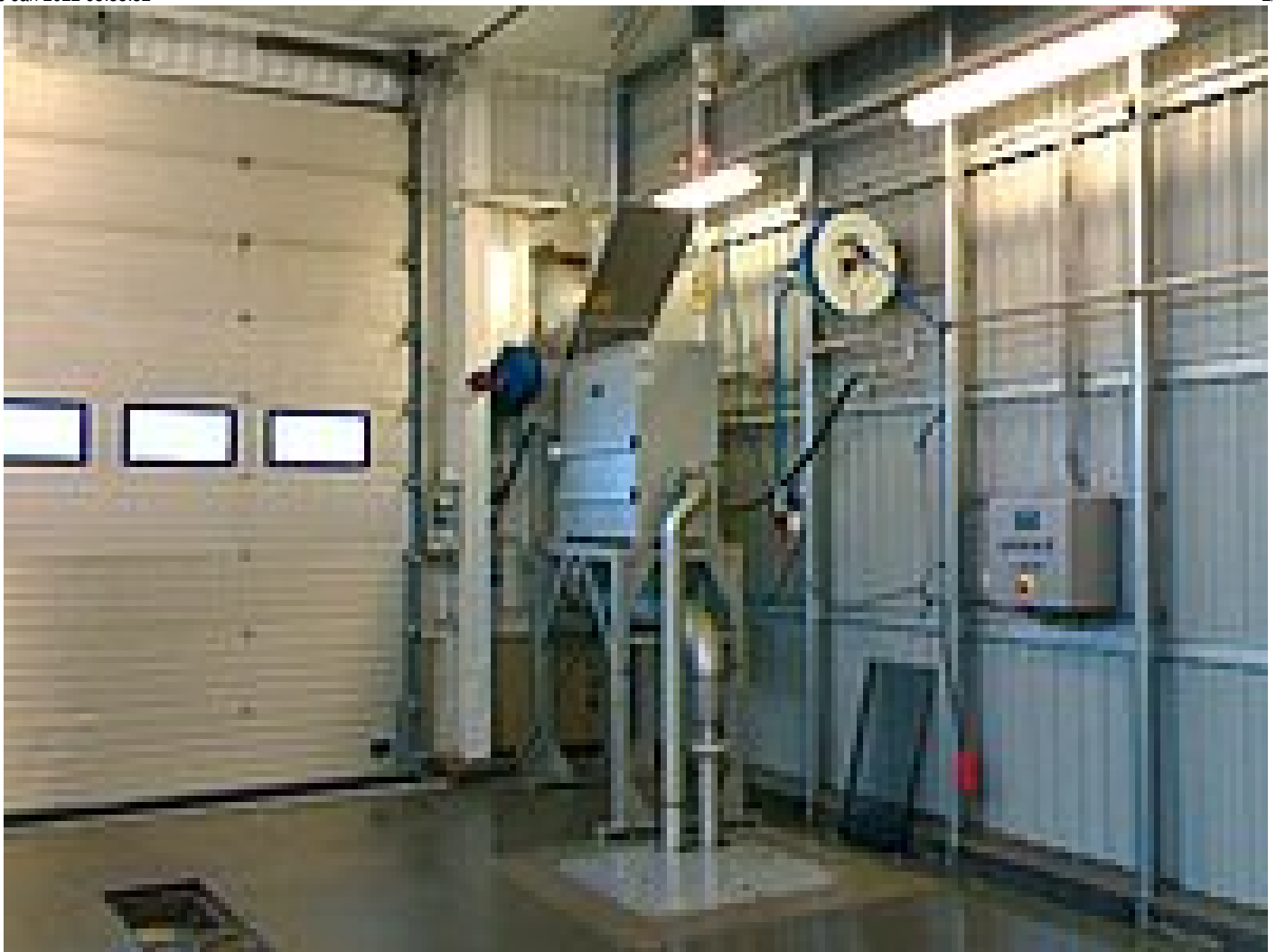
ROTAMAT® Ro 9 micro-strainer screening wastewater from livestock vehicle washing
