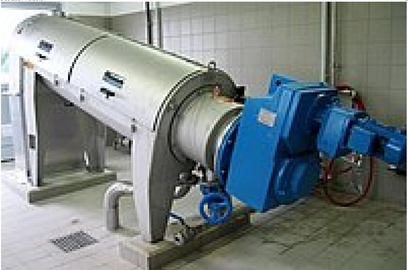
*The RoS 3Q 440 system is designed to dewater thin sludge with 1% DR or thickened sludge with 3% DR*
