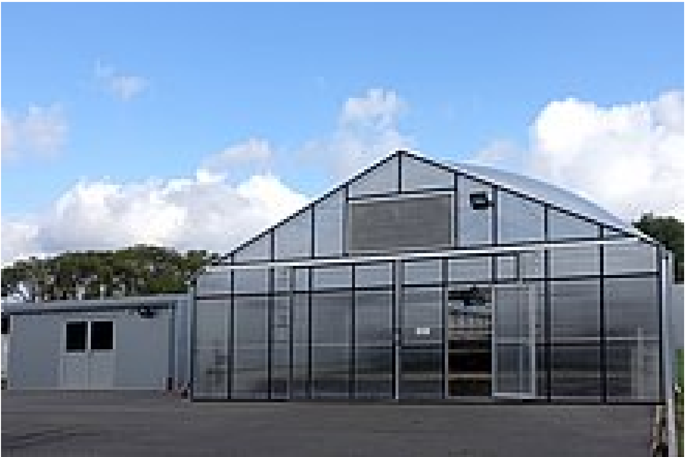
The sludge treatment plant is a completely automated, low-maintenance system
