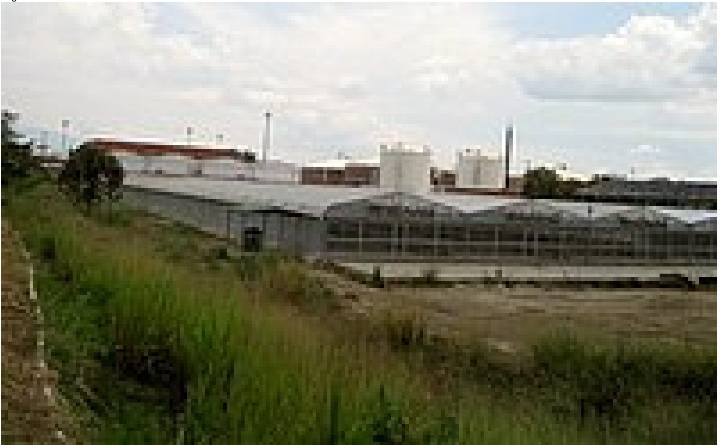
The sun makes sludge a valuable resource: The solar dryer at Cali produces fertilizer
