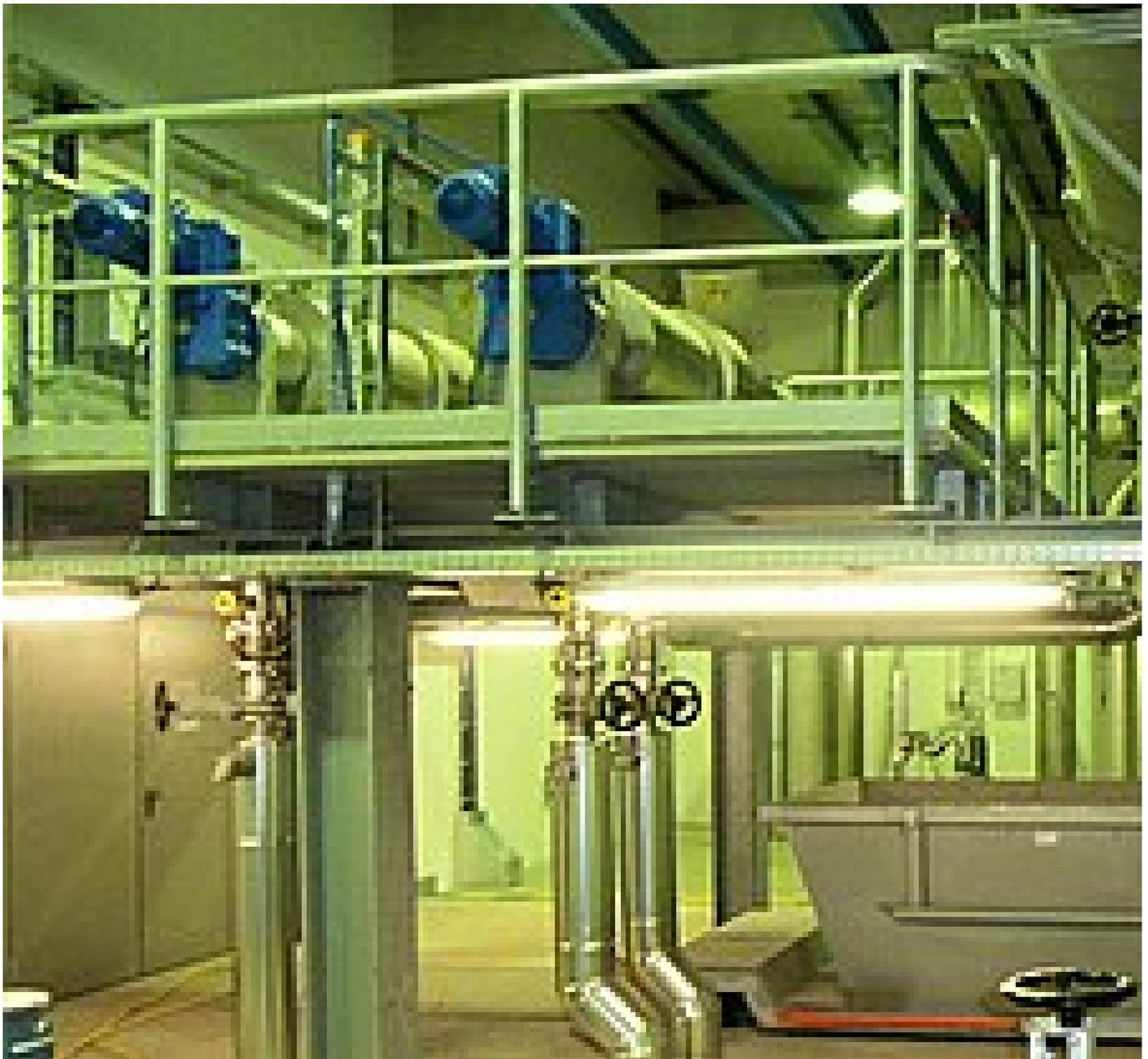
*Two insulated STRAINPRESS® machines for grease sludge screening, below a container into which the screenings are discharged*
