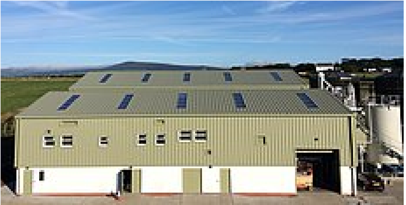
Exterior view of the drying hall
