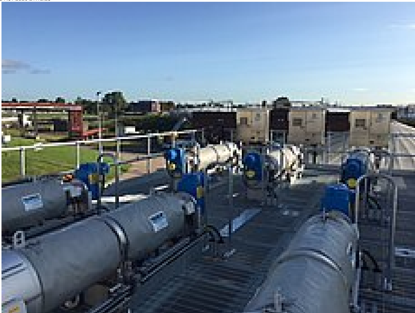
Minworth STW STRAINPRESS® Installation
