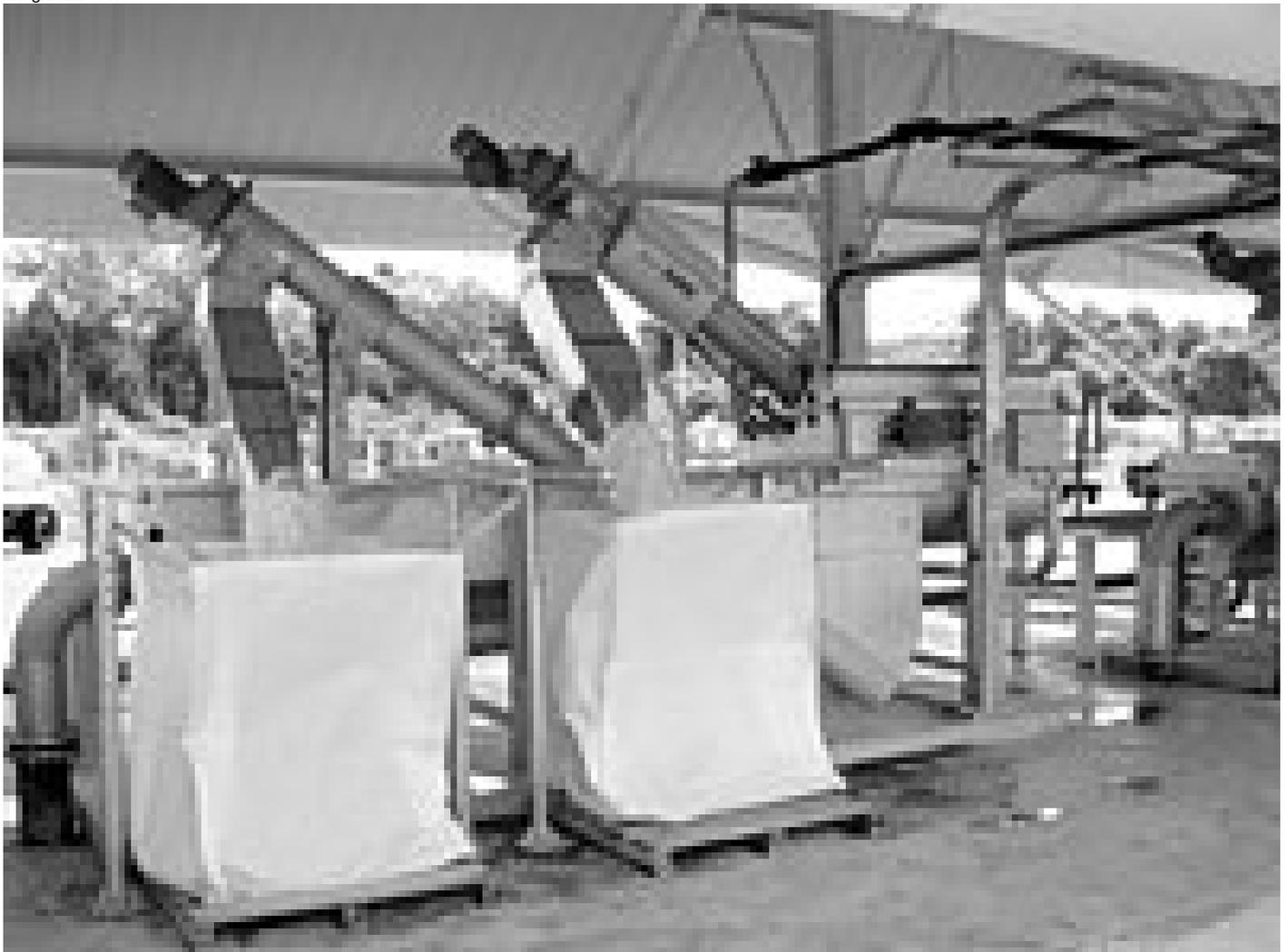
*Complete mechanical preliminary treatment: removal of screenings and grit by the HUBER ROTAMAT® plant*
