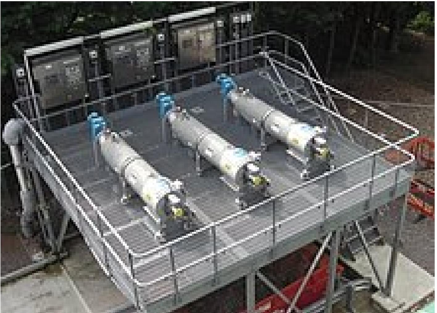
Figure 4 - Three STRAINPRESS® units installed on a platform, with control panels and frost protection fitted
