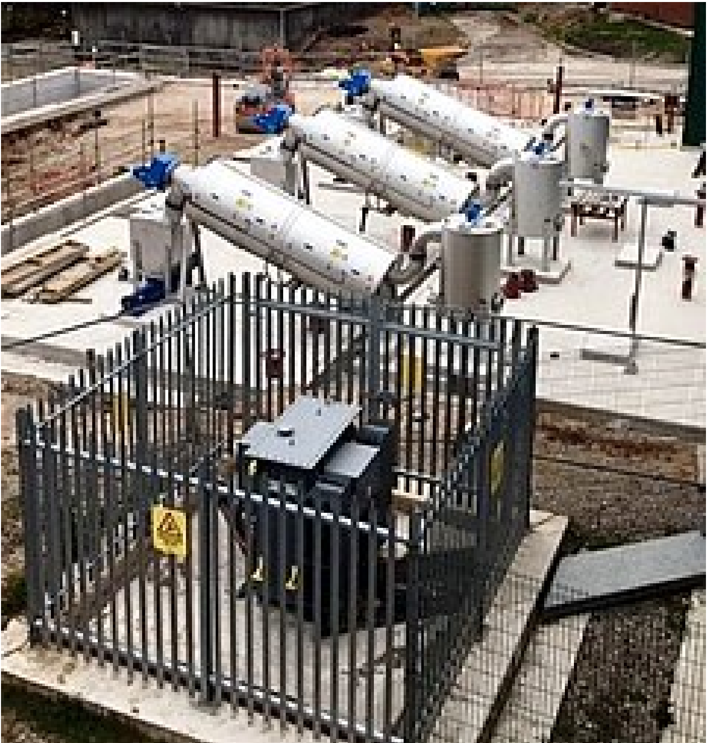
Photographs taken during the installation phase
