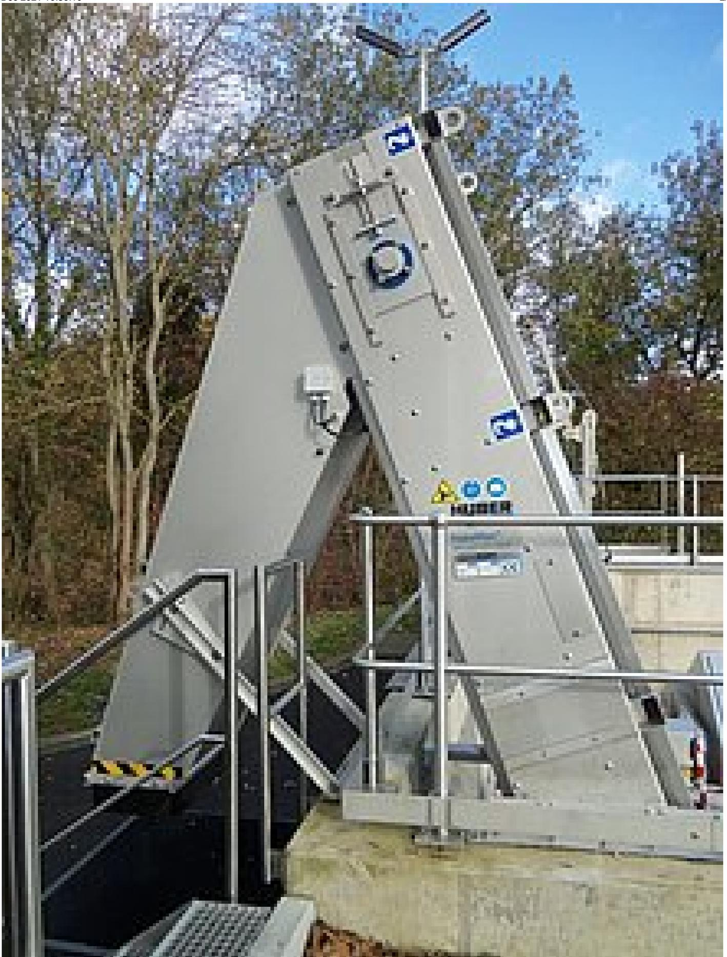
*In-channel installation of a RakeMax@-J screen on STP Aachen-Horbach*
