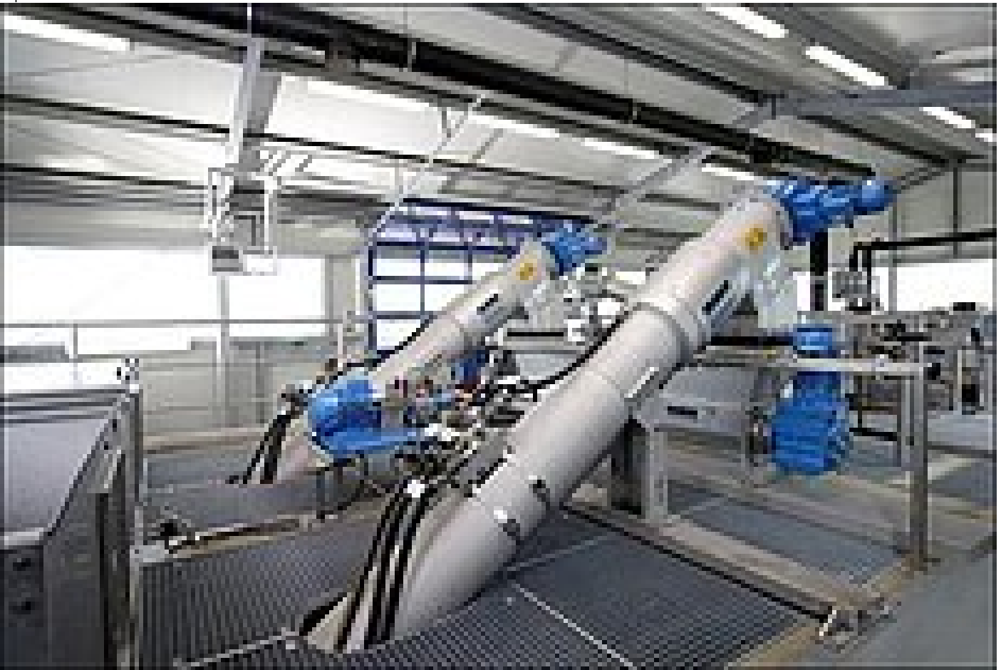
The coarse screen is a 5 mm STEP SCREEN®, the fine screen is equipped with a 1.0 mm mesh. The screenings from the fine screen are dewatered and discharged into a container
