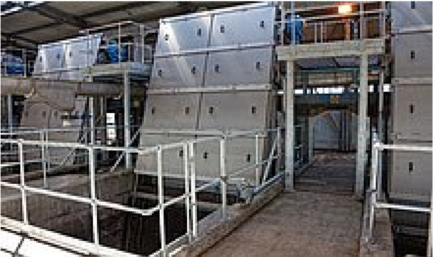
RakeMax® installation had to be completed through the roof of the building
