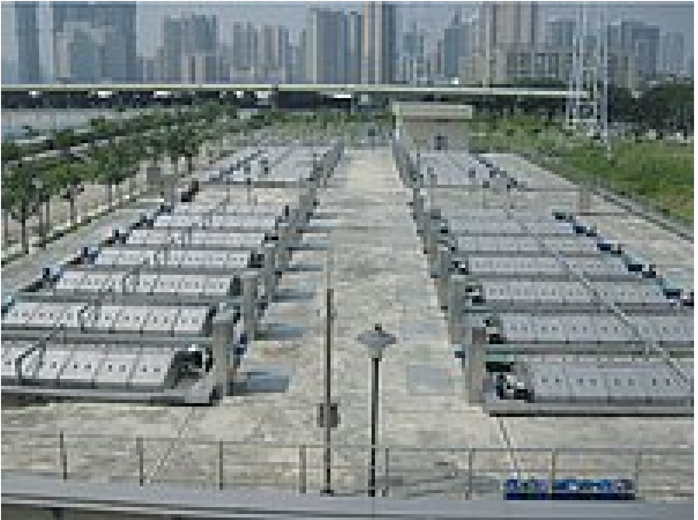
28 RoDisc® Rotary Mesh Screen units with 24 discs each treating about 8.5 m 3 wastewater per second
