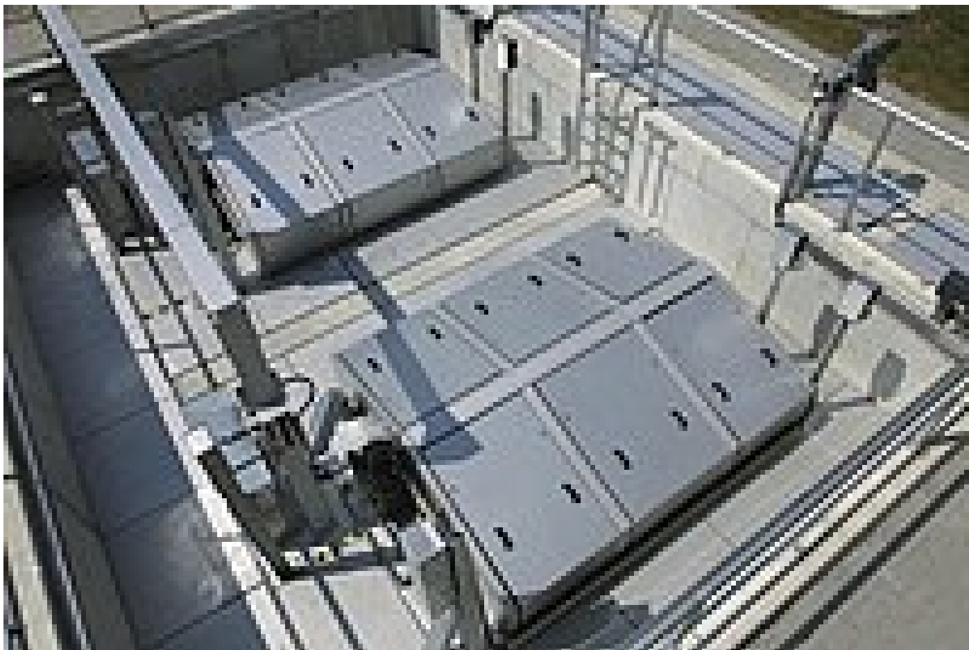
RoDisc® Rotary Mesh Screen for the retention of activated sludge flocks
