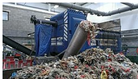
Drained and compacted rejects
