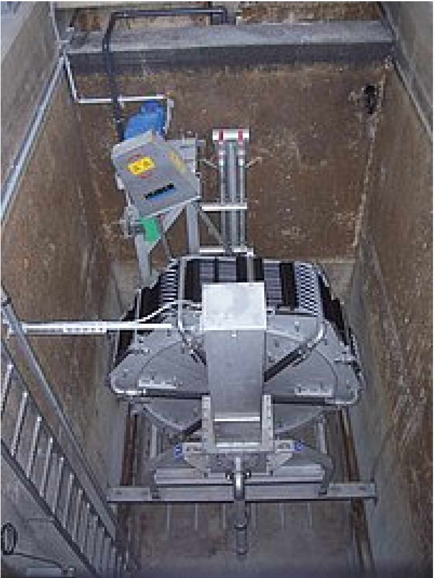
VRM@ 20/60 after installation
