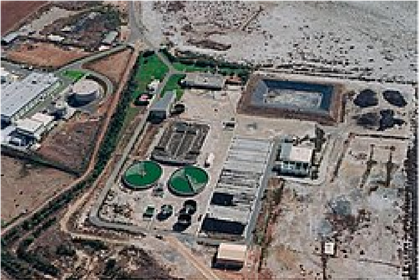
Sewage treatment plant Larnaca [image source: Google Earth]
