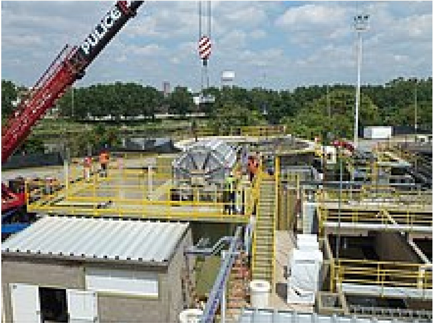
The two VRM@ 30 / 480 units during installation into the membrane chambers
