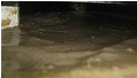
Organic material washed out ...
