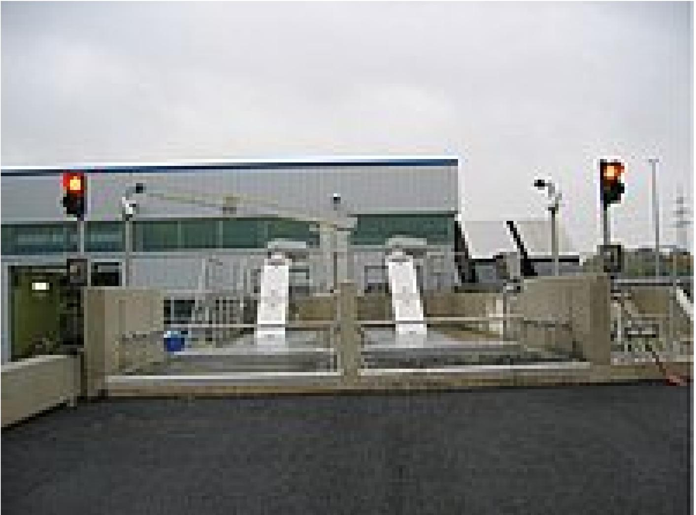
*Pair of 20 m<sup>3</sup> slurry receiving tanks with Ro 8 screw conveyors*
