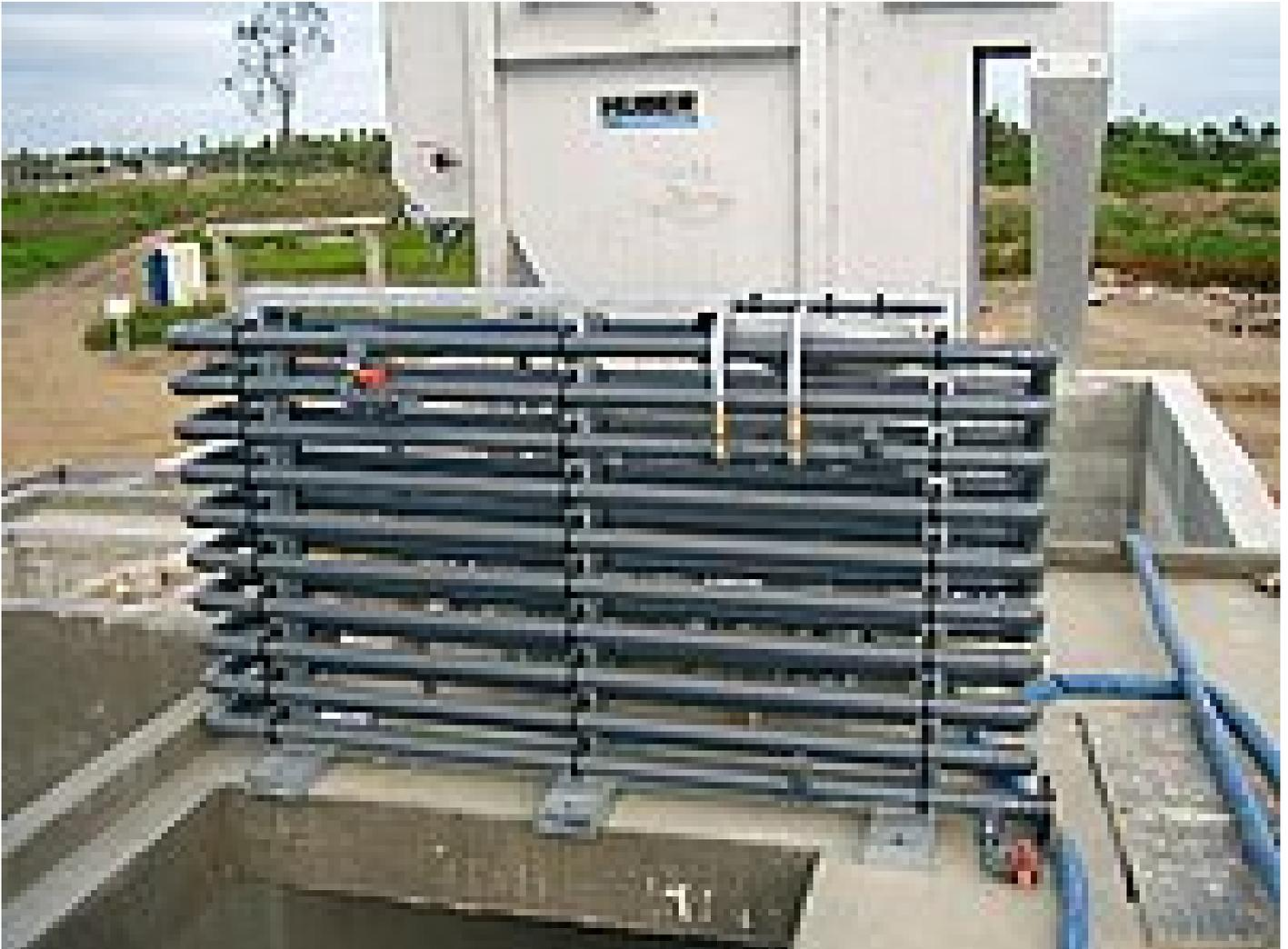
*Tubular reactor for chemical conditioning*
