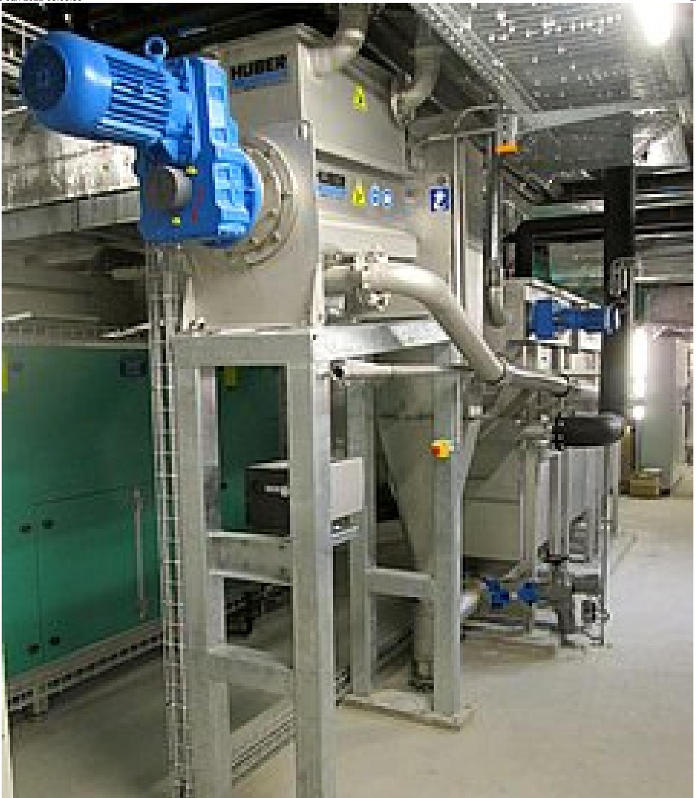
Fig. 2: Pre-screening (6 mm) of wastewater with HUBER Wash Press WAP®
