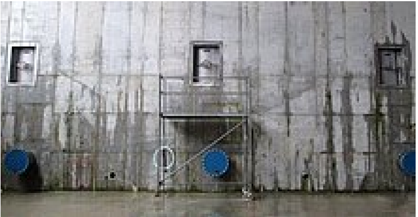
Fig. 2: The three TT7-30 pressure doors shortly after installation into the ozone reaction chambers at the Echthausen waterworks
