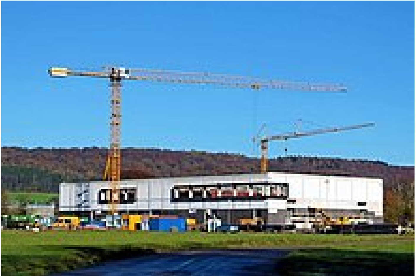
Fig. 1: Construction site of the new treatment building at Echthausen waterworks
