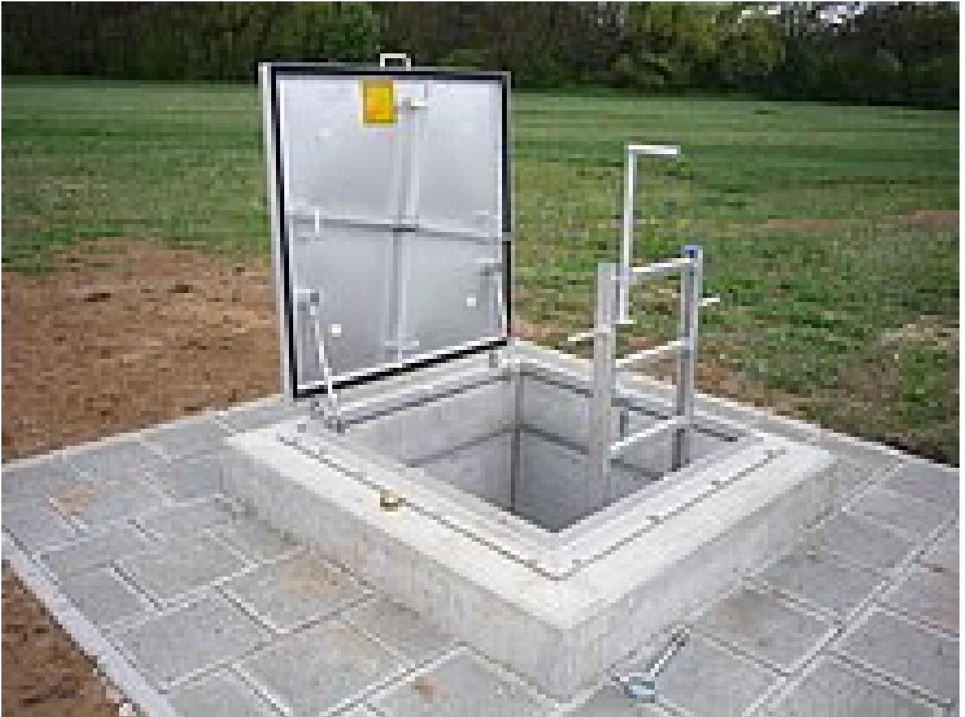
Newly refurbished manhole
