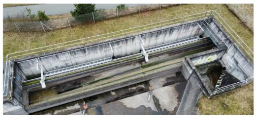
Fig. 28: A discharge structure with HUBER Storm Screen ROTAMAT<sup>®</sup> RoK1 TS that operates reliably even in heavy rain, combined with large amounts of screenings.
