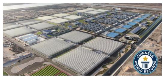
Fig. 44: Clean water for the Sinai Peninsula: The water treatment plant in Bahr El-Baqar (Egypt) has recently been awarded by Guinness World Records as the world's largest plant of its kind. More than two billion cubic meters of water are to be treated here annually on an area of about 650,000 square meters. Among other things, HUBER supplied 128 SOSLTICE<sup>®</sup> sludge turners to dry 490,000 tonnes of dewatered sludge annually with the help of the sun.
