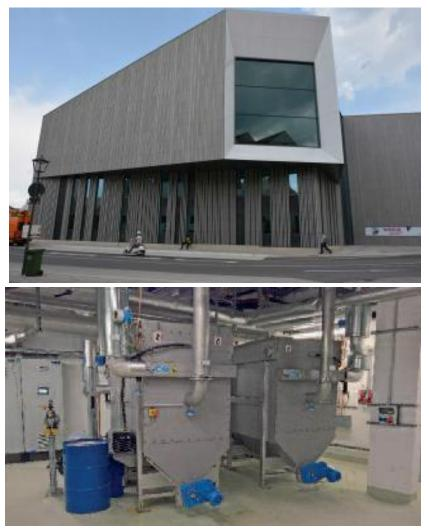
Fig. 31: Wastewater heat utilisation – the Museum "Haus der Bayerische Geschichte" (pictured above) in Regensburg uses the HUBER ThermWin system with the HUBER Heat Exchangers RoWin (pictured below) to heat and cool the building. This replaces fossil fuels with renewable wastewater energy.
