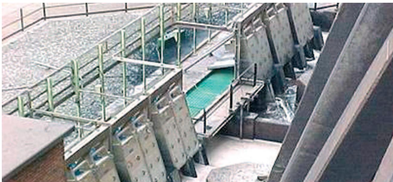
*Seven HUBER STEP SCREEN® Vertical units installed in the inlet to the cooling tower*
