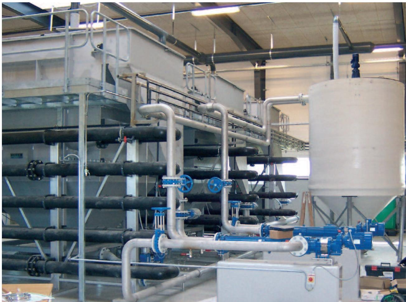
*HUBER Dissolved Air Flotation Plant HDF 7 with chemical treatment stage and sludge tank*
