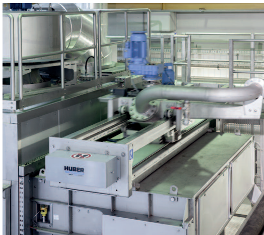
HUBER Extruder for feeding the dewatered sewage sludge
