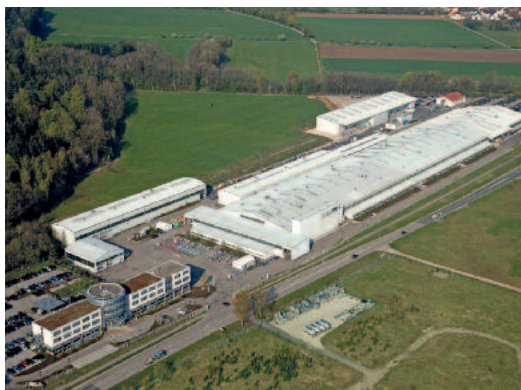
The HUBER SE company site in Berching / Erasbach
