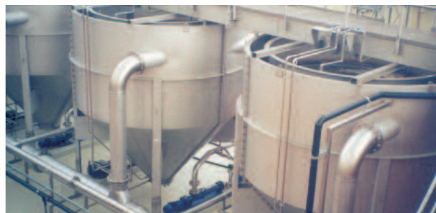
HUBER Circular Grit Trap HRSF installation
