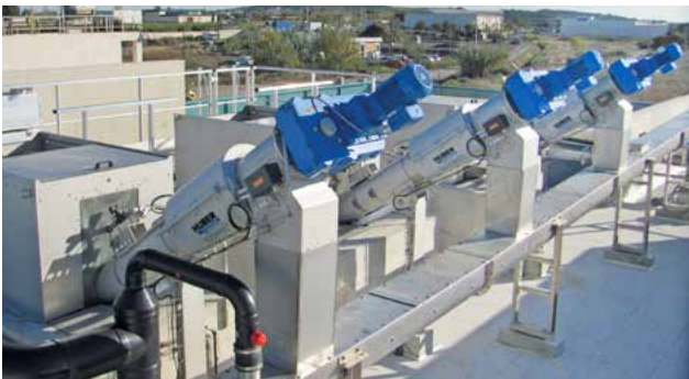
3 ROTAMAT® STAR units size 1000 with 1.5 mm perforation protecting the downstream membrane plant.
