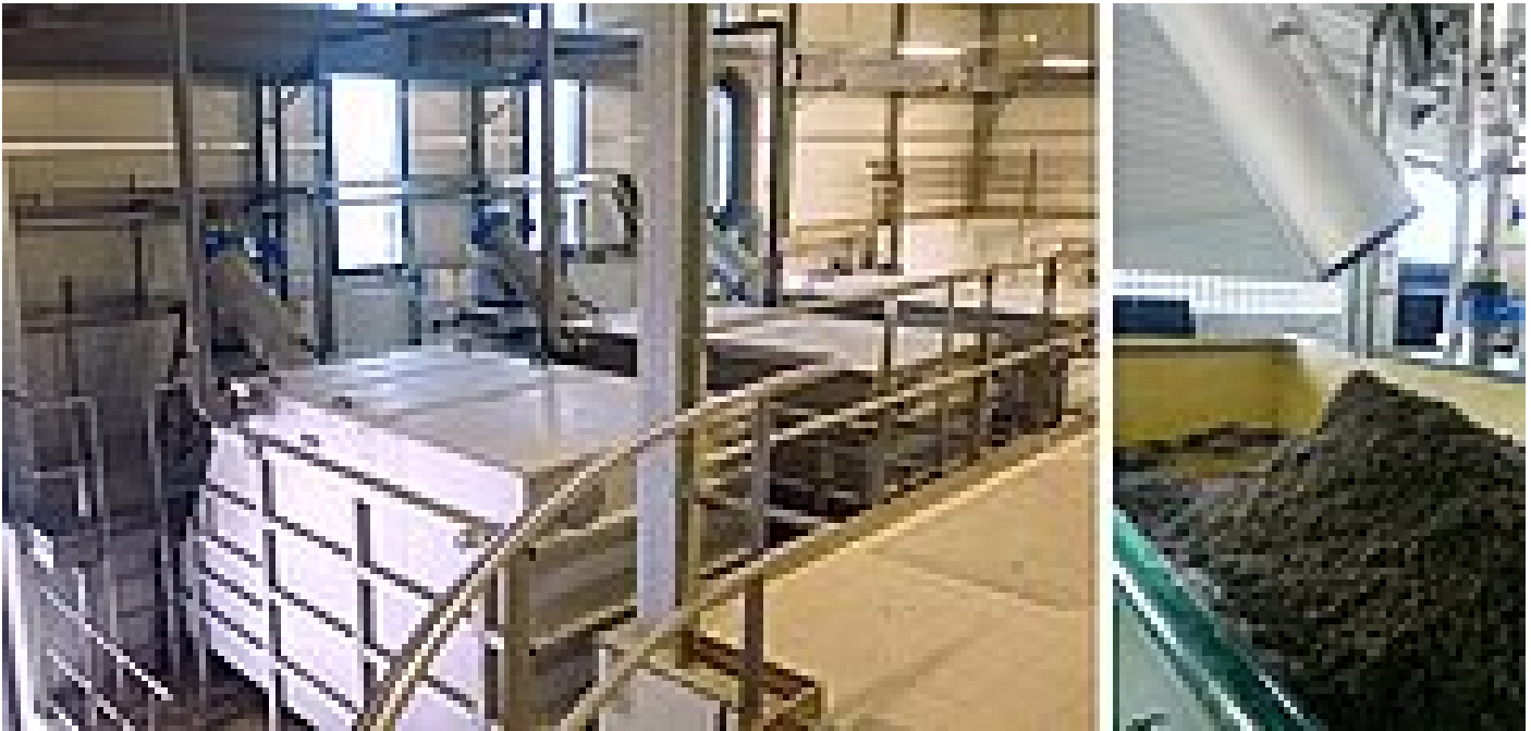
Fig. 1: Fine Screen HUBER ROTAMAT® STAR with a throughput capacity of 1.000 m 3 /h each providing excellent dewatering results of > 35 % DR
