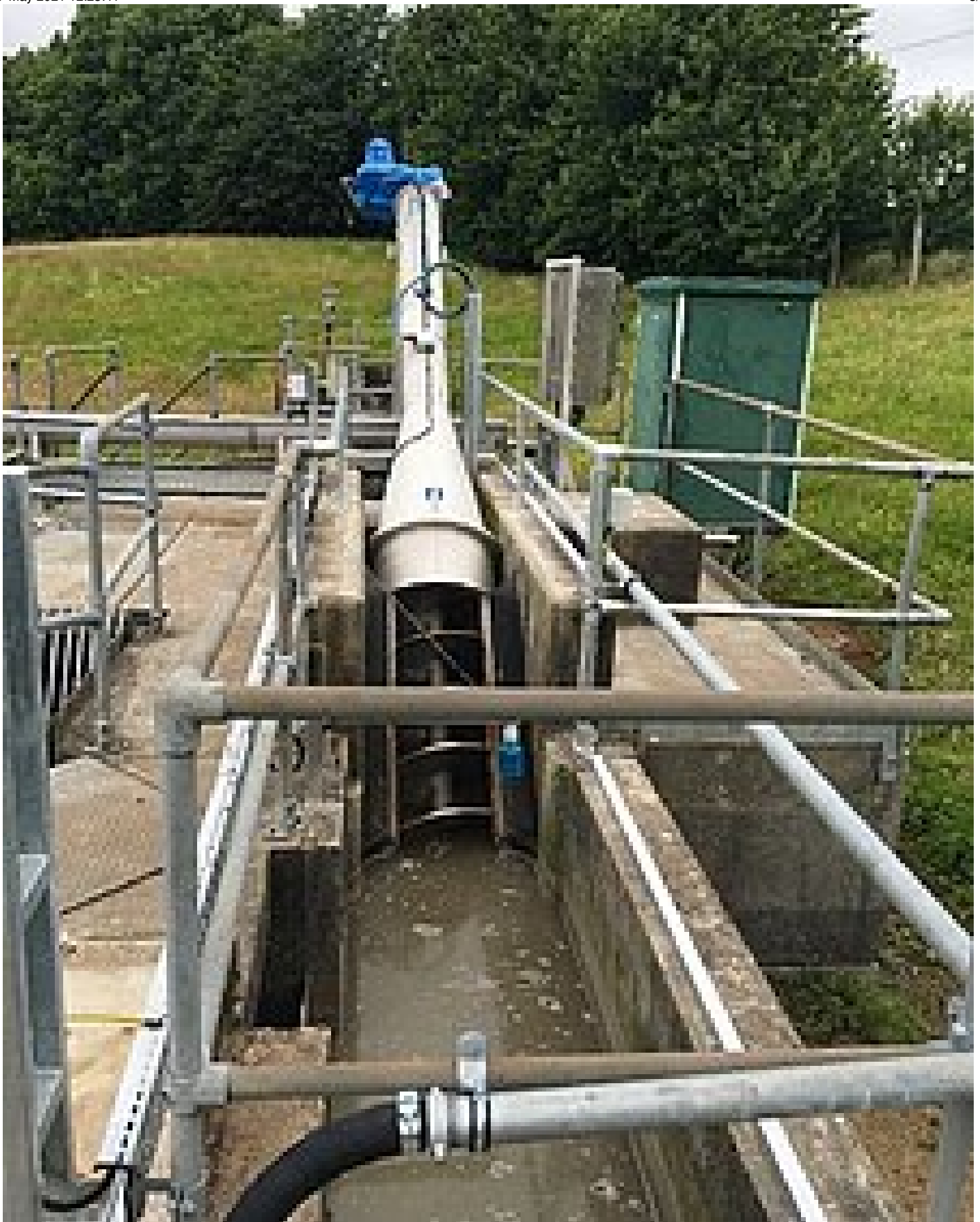
The modified HUBER Micro Strainer ROTAMAT® Ro9 in the inlet screen channel
