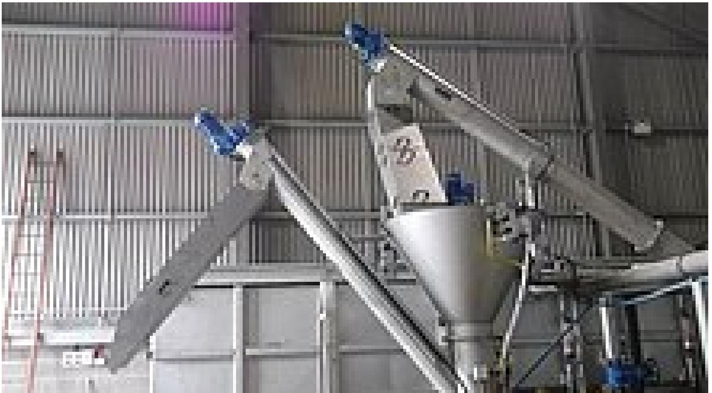
*Grit washer was elevated so that the overflow drained back to the grit trap*
