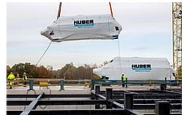
*After the dryers have been lifted into place, the steel construction above the dryers can now continue*
