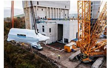
*The dryers are lifted directly into the building onto the prepared level*
