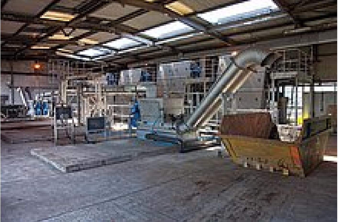
Huber Technology has completed the upgrade of the inlet works at Meadowhead STW. The project involved the installation of 4-off HUBER RakeMax® Multi-Rake Bar Screen 6300/2752/19 Coarse Screens and 2-off 12 m<sup>3</sup>/hr HUBER WAP-L Wash Press Screening Handling units for the Coarse Screens and 2-off 15 m<sup>3</sup>/hr WAP-L Wash Press Screening Handling units for the retrofitting into the existing inlet works for handling screenings from the Fine Screens.
