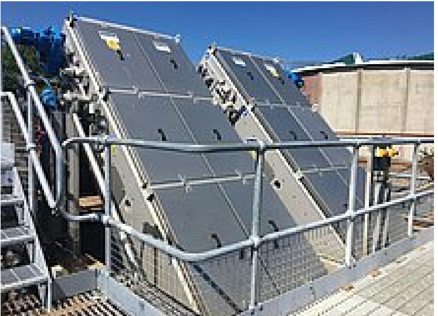
New EscaMax® screens installed at 60 degrees into the existing inlet works
