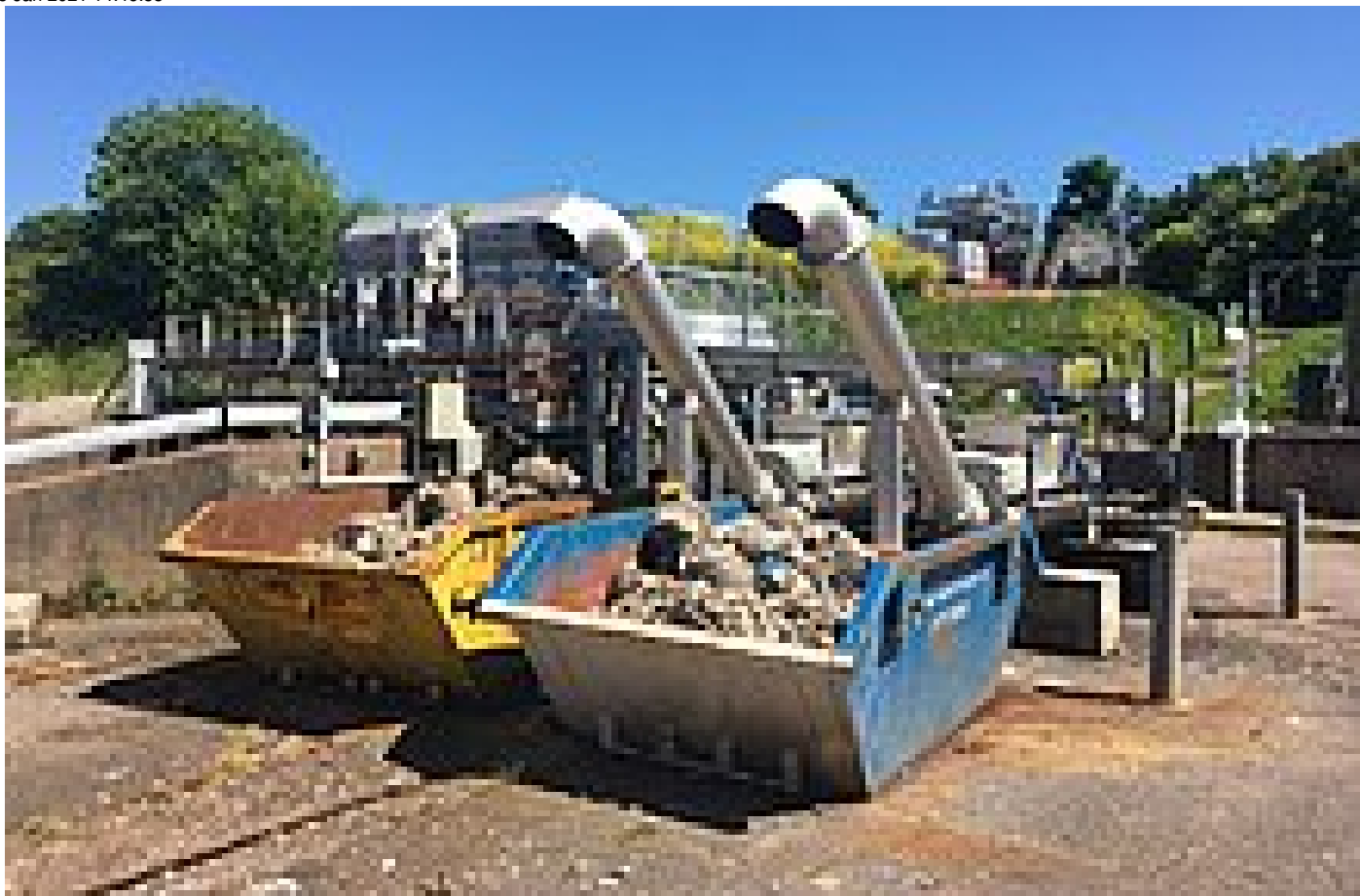
New HUBER Wash Press WAP®-L BG4v screenings handling plant, EscaMax® inlet screens and RakeMax® bar screen in the background
