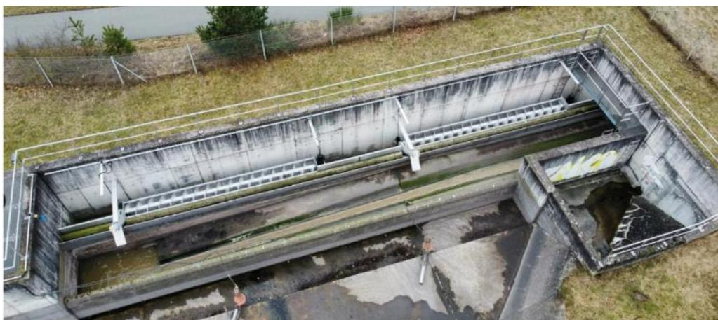
Fig. 28: A discharge structure with HUBER Storm Screen ROTAMAT® RoK1 TS that operates reliably even in heavy rain, combined with large amounts of screenings.
