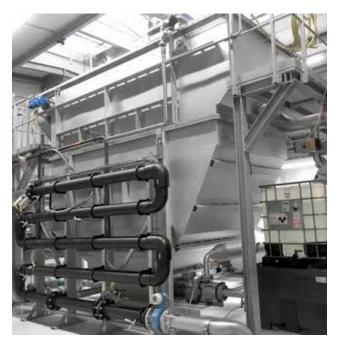
HUBER Dissolved Air Flotation Plants with chemical pre-treatment – full, partial or secondary treatment of industrial wastewater
