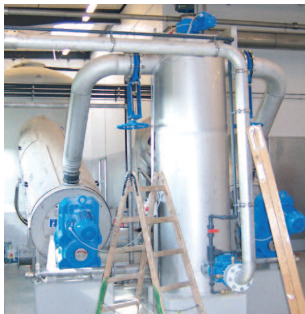
Flotate sludge dewatering with two ROTAMAT® Screw Press RoS 3/3 units with pipe reactor during installation
