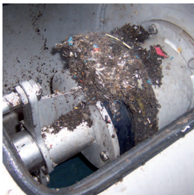
Removal of dewatered disturbing matter from the material separator
