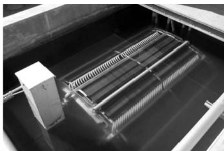
From the top of the vacuum rotation membrane's filtration tank, it is obvious whether the unit's air scouring is on (left) or off (right).
