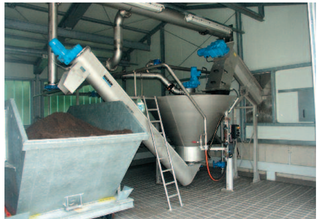
COANDA Grit Washer for improved hygiene and reduction of disposal costs
