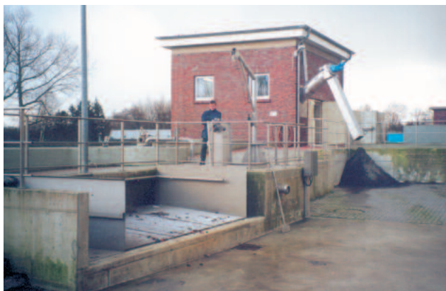
The RoSF 5HP system allows for long distances between the tank and Grit Washer.
